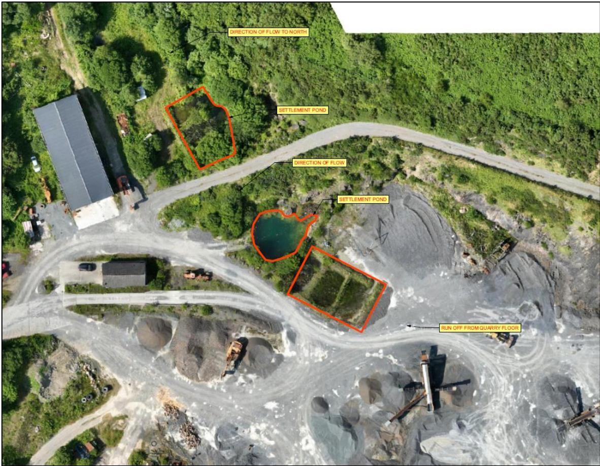
Figure 7.8 - Existing Ponds & Discharge Point
