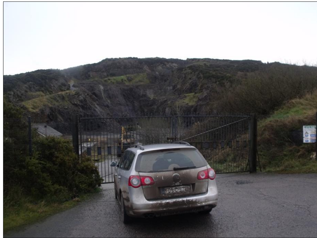
Plate 1 Front entrance of existing quarry. Looking east towards Ardkill More upland.
