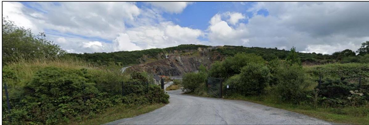
Photograph 2.4 – View of Existing Entrance to the Site
