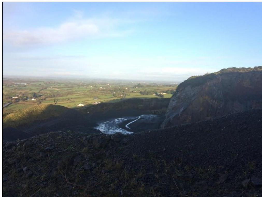
Plate 2 Looking north-west showing haul road within quarry.
